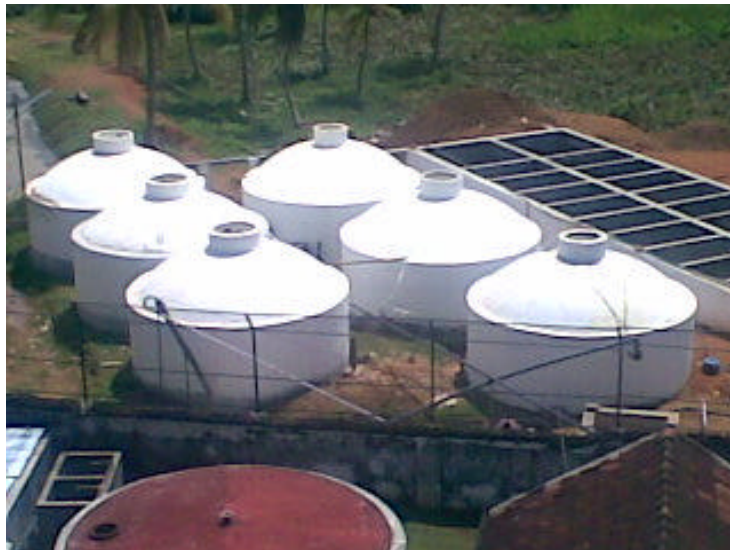
Fig. 2 Wastewater treatment system (according to Anaerobic filter technology UAFF) of Sri Lanka Distilleries ltd. - Wadduwa distillery, Sri Lanka
